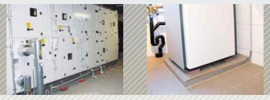
Air conditioning (AC) systems bedded on Isotopo SE elements. Sylomer® discrete bearings for a heat pump
