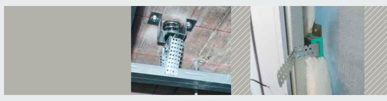
Spring hangers for suspended ceilings with a low natural frequency
